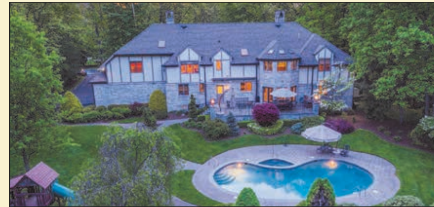
Saddle River: Elegant updated Tudor style estate, this "Smart Home" is majestically set behind gates on beautiful grounds in one of the most sought after neighborhoods! Double front doors lead to a grand 2 story entry foyer with coffered ceiling, 2 story great room with 23 ft. stone fireplace, coffered ceiling and full bar. Incredible master suite with fireplace, sitting room, 2 walk in closets, & spa like bath. Also boasts home theater, gym, music room, gaming area, 900 bottle wine cellar, heated gunite salt water pool with spa, tennis & basketball court. $2,995,000
